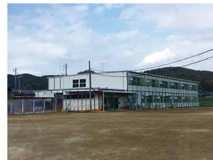
▲ Temporary building of Kawabe Elementary School in the ground of Sono Elementary School (Source: CWS Japan, November 9th, 2018)
