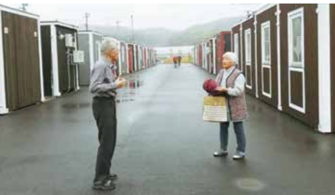
▲ Prefabricated temporary shelters in Yanaihara area (Source: 豪雨ニモマケズ)
